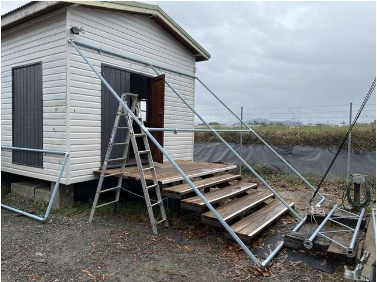
Fitting of the canopy frames underway
