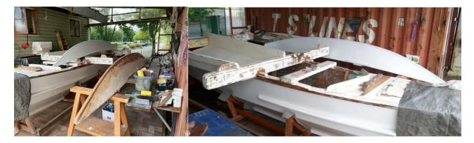
Seating has been altered and trimmed in anticipation of the crossbeam conversion. The major work underway is Phill leading the team to produce a bird's beak join fabricated 5.5 metre mast from Northern Sassafras. Lots of effort, tense moments, cross words and teamwork to find the timber, machine into strips, cut, assemble, glue and plane the glued product into a round mast ready for sanding.
