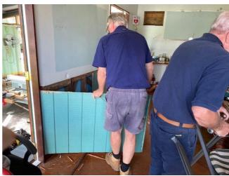
The rear wall was stripped bare of everything but the kitchenette, and so was the side wall betwixt the two double doors. It was all trimmed as flat as possible – not an easy task with such an old, transportable building – and then both areas re-sheeted with plasterboard.
