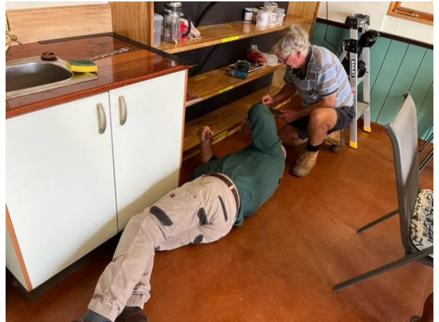
Painting & clear-coating complete, installing shelf braces.
