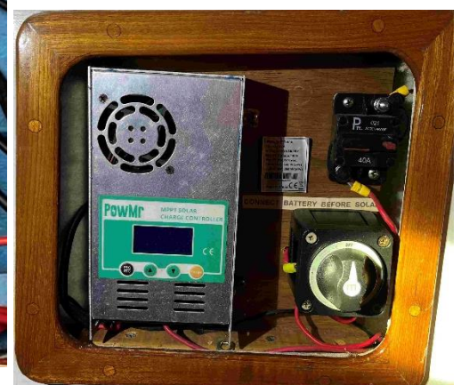
Solar charge controller with newly installed 3-position switch
