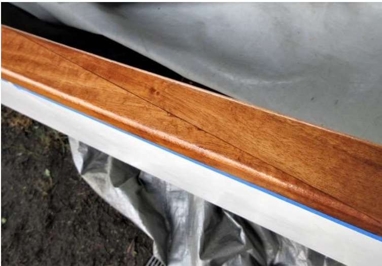
A nice photo of a scarph, varnished:
