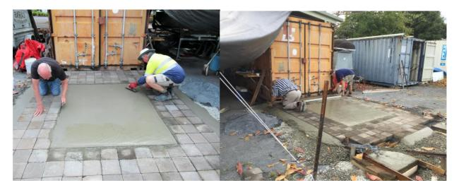
You can see in the above right hand shot that the container footings have heavy chain inserts for securing the containers. We have duplicated the original footings in this case.
